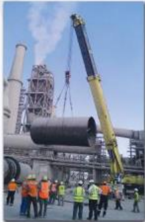
Lifting for Kiln Section
