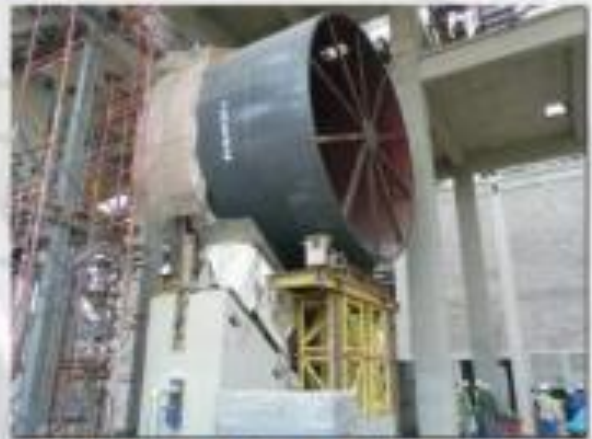
Erection of Cement Mill section
