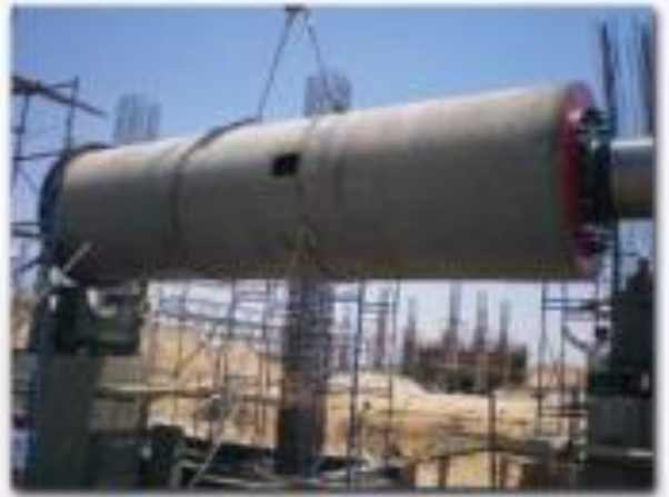
Erection of Cement Mill
