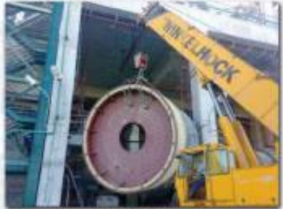
Erection of Cement Mill Section
