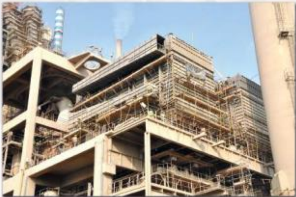
Erection of Raw Mill A & B Bag Filter - TOURAH Plant II Line 8 - 2011-2012
