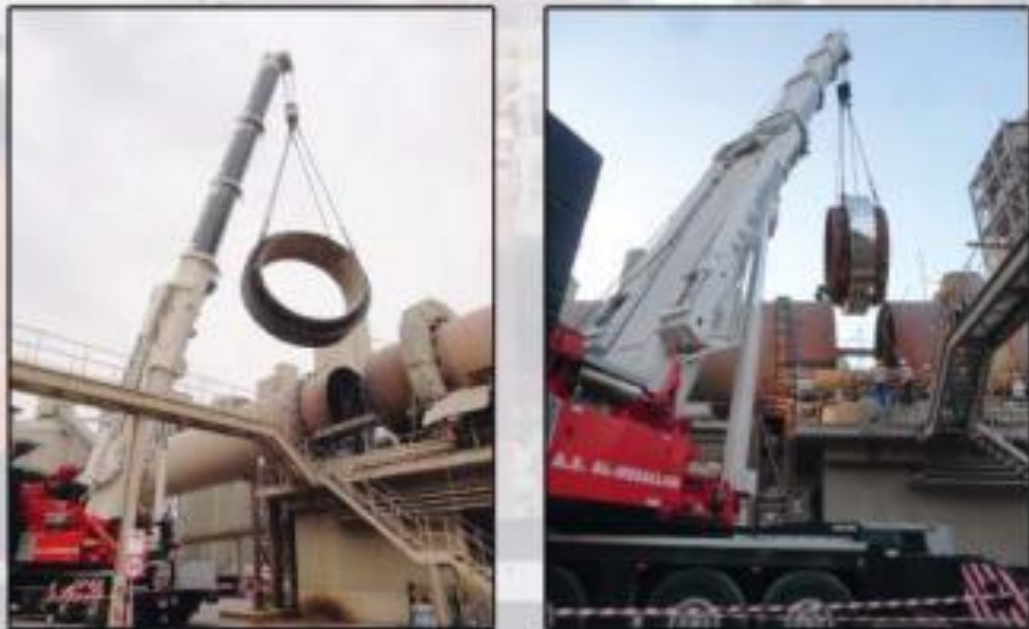
Yamama heavy Section Replacement
