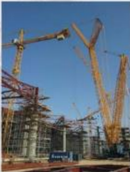
Erection of 2200 tons Steel Structure King Khaled international air port ( terminal 5 )
