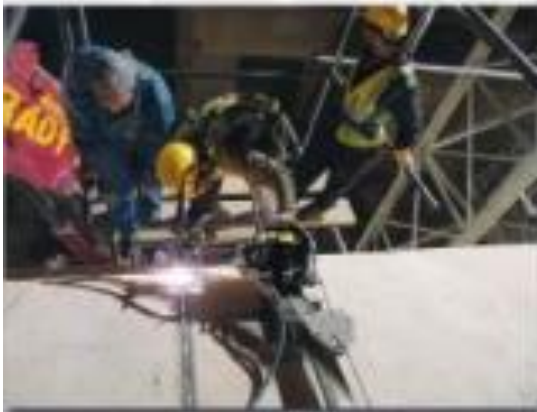
Cutting of Kiln Section - TOURAH Plant II Line 9 - 2010
