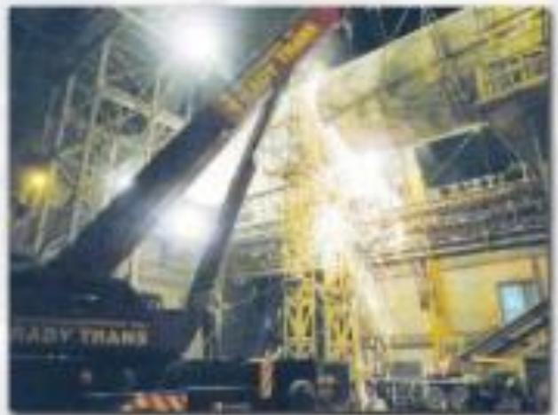
Replacement of Kiln Section - TOURAH Plant II Line 9 - 2010
