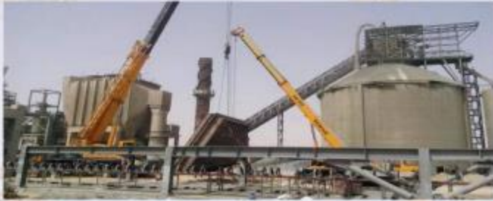
Erection of vertical cement mill and packing at El-Sewdy Cement Company
