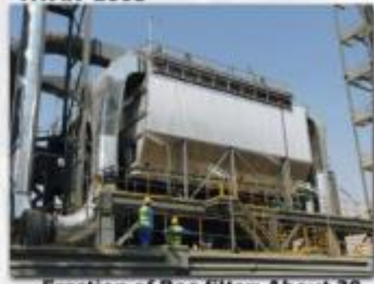
Erection of Bag filter; About 30 filters was erected in Arabian Cement Line II - 2010
