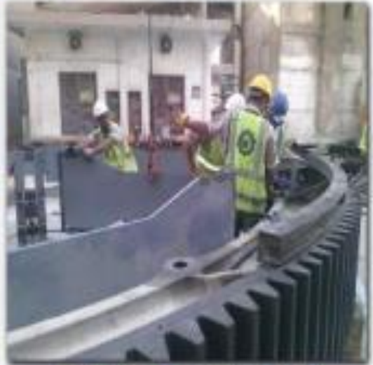
Girth Gear assembly work
