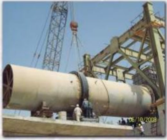
Erection of Kiln.
