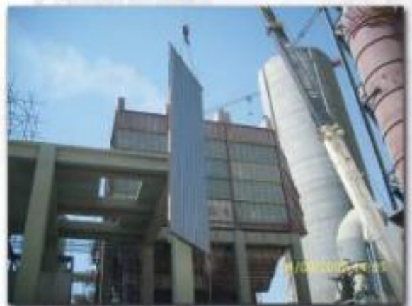
Erection of Collecting plate
