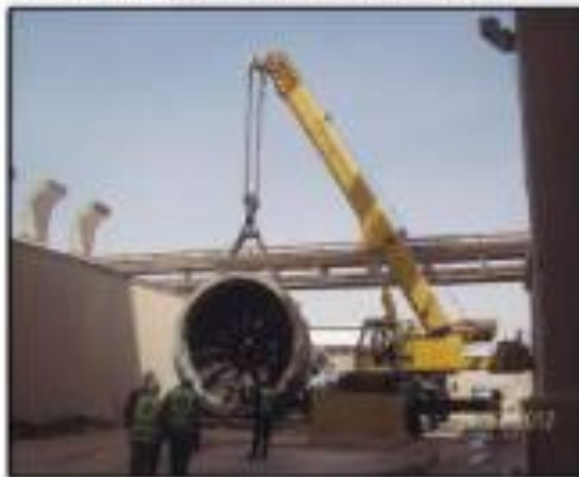
Loading the Raw Mill Section
