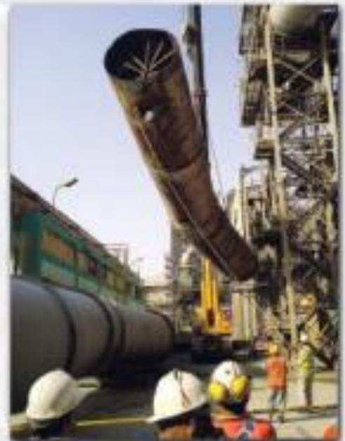
Replacement of Tertiary air duct TOURAH Plant II 2011
