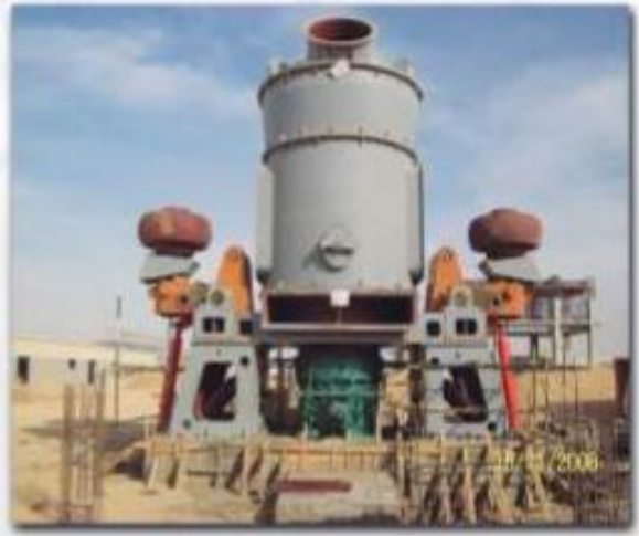
Erection of Vertical Mill.
