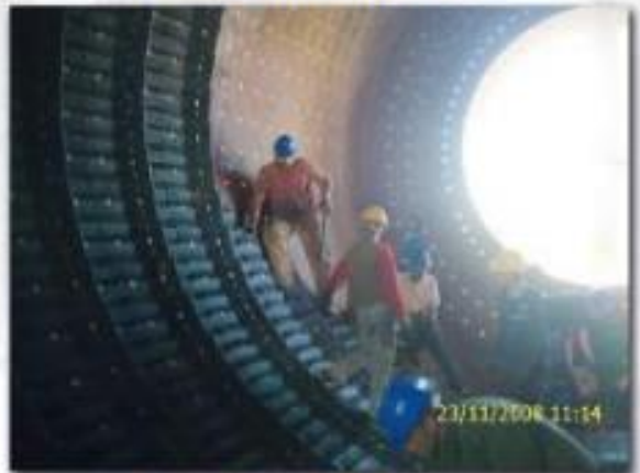
Erection of Mill liner
