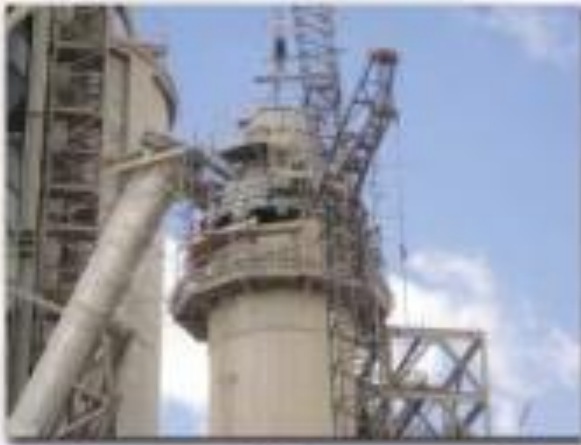
Replacement of inlet cone and inlet bend for bypass GCT - NLS in ACC II 2012
