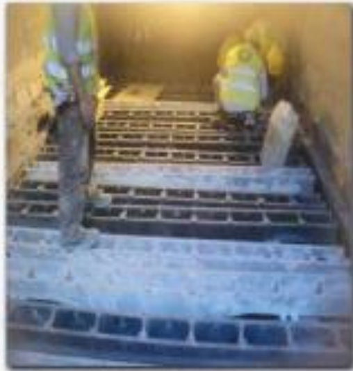
Replacement of Cooler Liner and adjusting
