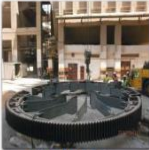
lifting of girth gear
