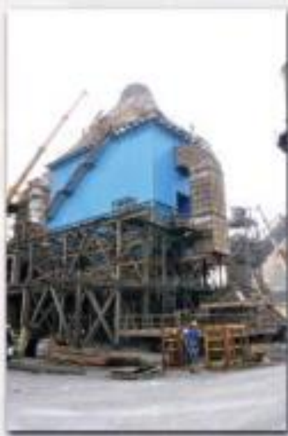
Erection of Bypass, Clinker Cooler, Raw Mill A & B Bag Filter TOURAH Plant II Line 8 - 2011-2012
