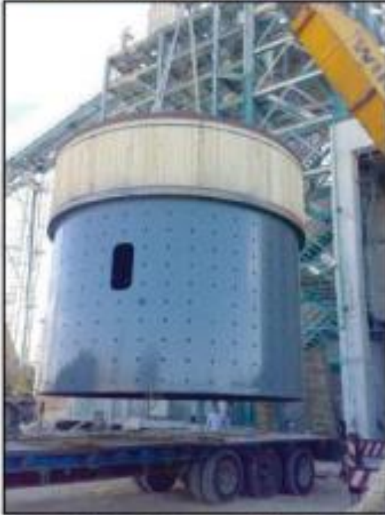
Unloading of Cement Mill Section
