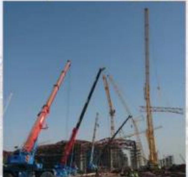
Erection of 2200 tons Steel Structure King Khaled international air port ( terminal 5 )
