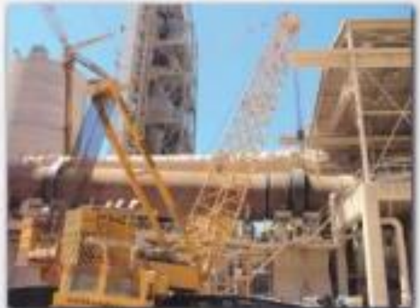
Replacement of Kiln three heavy section Zilten - Libya - 2010
