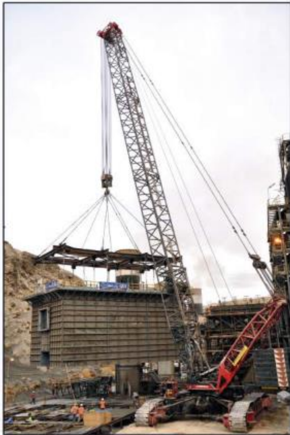
Lifting of Cooler Bag Filter
