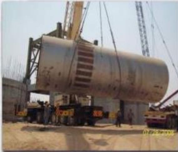
Unloading of Kiln Section
