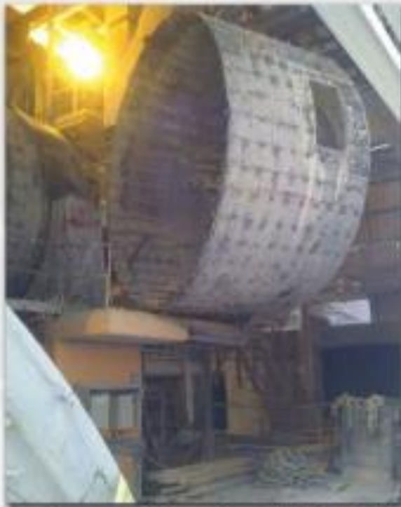
Replacement of sections in Raw Mill A & B TOURAH Plant II Line 8 - 2011
