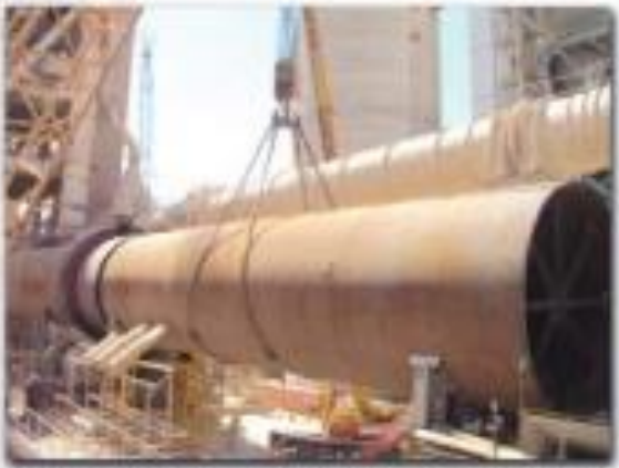
Replacement of Kiln Section - Libya -2010
