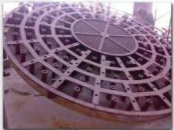
Erection of Diaphragm
